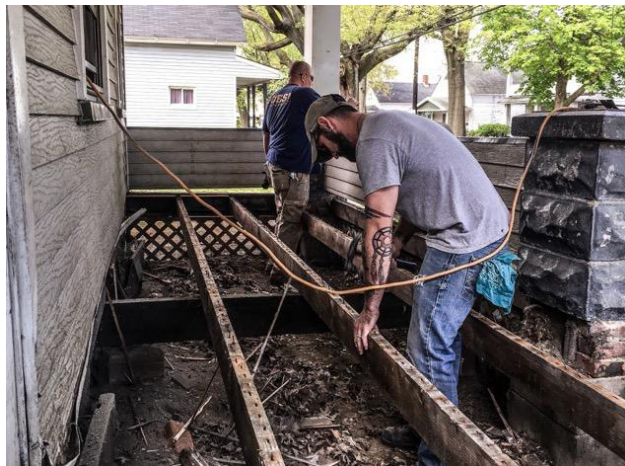
Repairing homes at Slavic Village, Cleveland.
